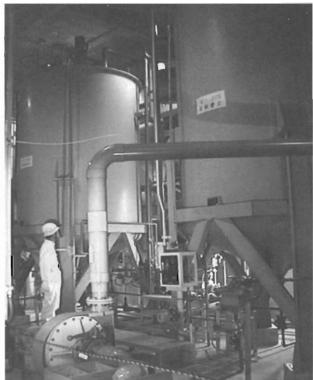
Photo 2 Large Tanks before Dismantling
