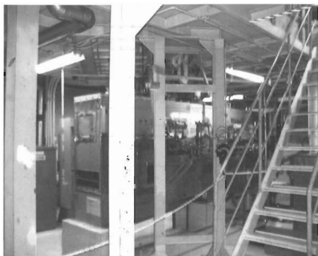
Photo 3 UF 4 Vacuum Filter Equipment before Dismantling
